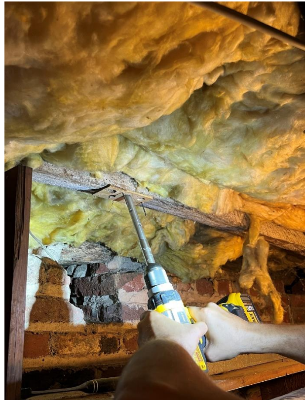
Dr. Daniel Miles extracts a core sample from an historic framing timber in the Belmont cellar. [Oxford Dendrochronology Lab photo.]
