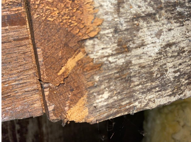
Floor joist, Belmont basement, photographed in May 2023 by Michael Spencer.
