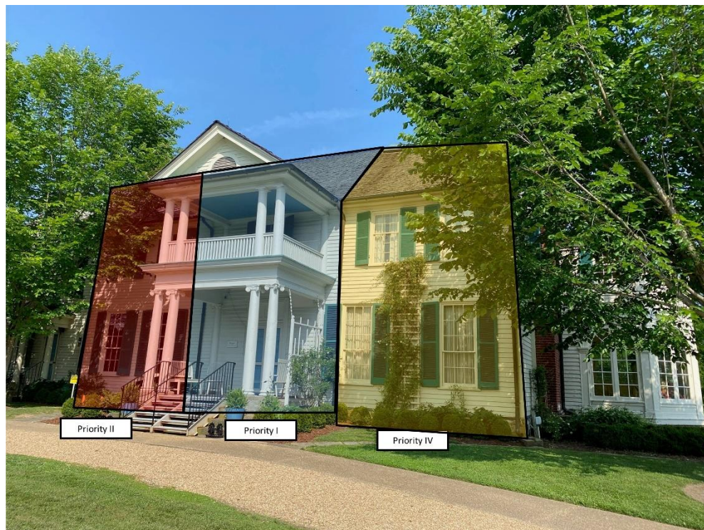
Belmont northwest elevation showing priority areas for dendrochronological investigation, prepared by Michael Spencer.
